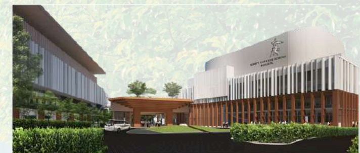
2024 CIB INTERNATIONAL SCHOOL 2500 KVA 2 SETS
