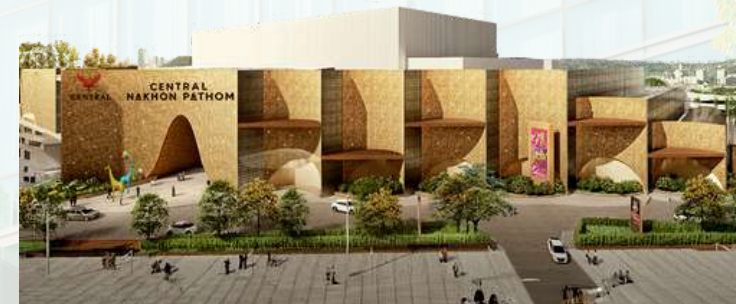
2023 CENTRAL DEPARTMENT STORE NAKHON PATHOM 1000 KVA 2 SETS
