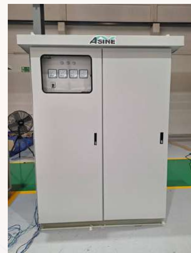
MDB Outdoor 400V 800-1600A = 2 panels W1600xH2275xD1000mm.
