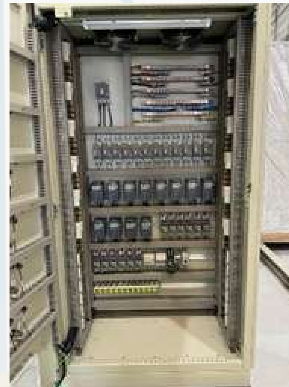
MCC Outdoor 400V 40A = 2 panels W1000xH1900xD600mm.
