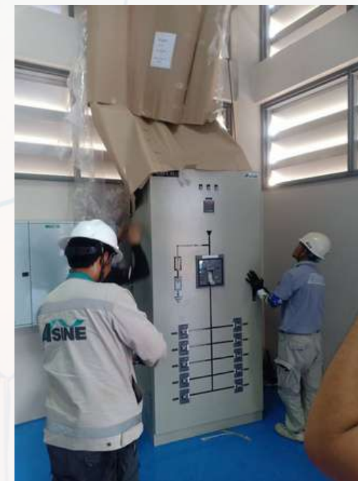
Motor Panel Indoor 400V = 1 panel W600xH1200XD300mm.
